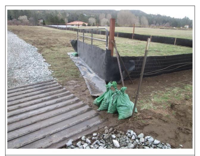
**Photo 2:** At the recommendation of the authorized biologist, arroyo toad protective measures for exclusionary purposes, such as the use of silt fencing around the yard and a rubber flap and gravel bags at the yard entrance, were observed being implemented at Creekside Staging Yard (Section 2.11 - Streambed Alteration Agreement).
