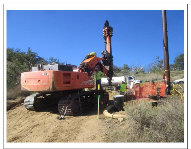
**Photo 3:** A drilling crew was observed repairing a hydraulic fluid leak on a drill rig and conducting stained soil cleanup. Absorbent pads and drip pans were observed being utilized, and stained soils were placed in a drum for disposal in accordance with the Spill Response and Notification Plan and MM-PHS-2.
