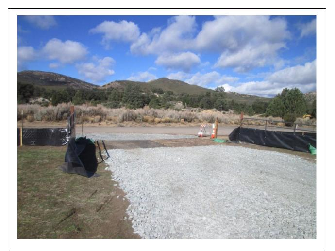
**Photo 4:** Track-out control BMPs, such as rattle plates and a rock apron were observed at the ingress and egress of Creekside Staging Yard in accordance with the SWPPP, Erosion Control Plan, MM-HYD-1, MM-BIO-7, and APM-HYD-09.
